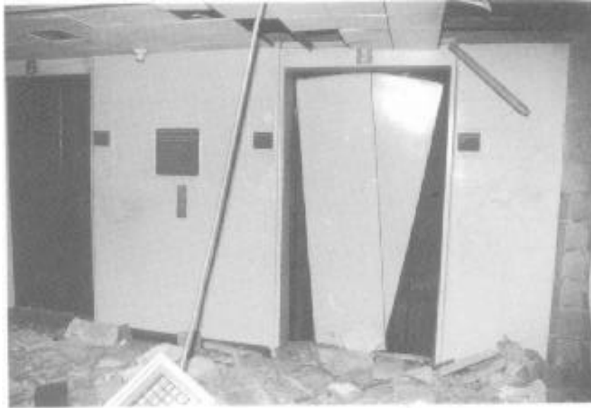
Damaged elevator doors and enclosures on the B-2 level presented a vertical channel for smoke spread into Tower 1. (Photo courtesy of Port Authority Risk Management.)
