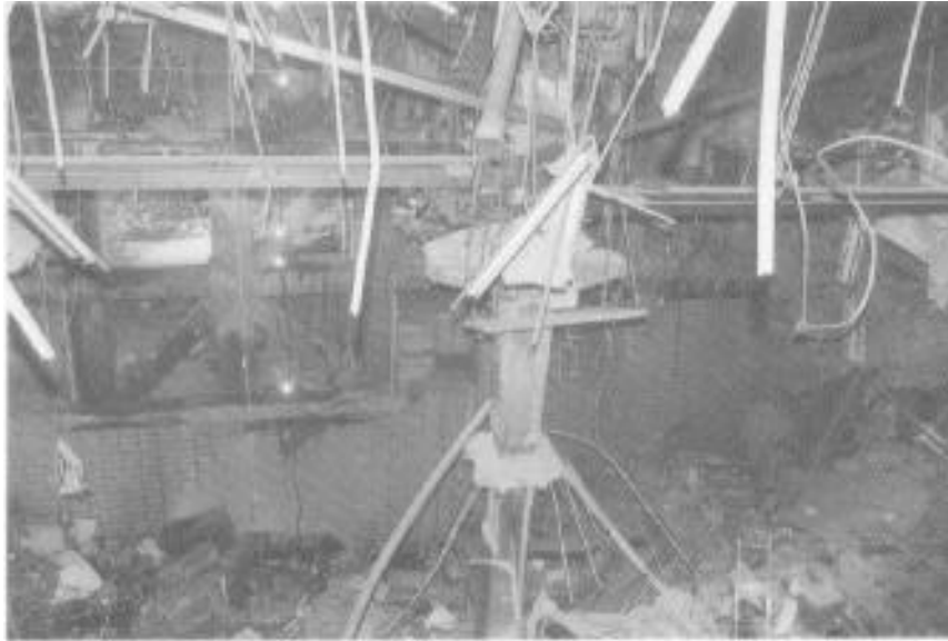
A view of the crater from the B-1 to B-5 levels. Note the steel column. Horizontal supports were destroyed in some cases, but the columns did not give. (Photo courtesy of Port Authority Risk Management.)
